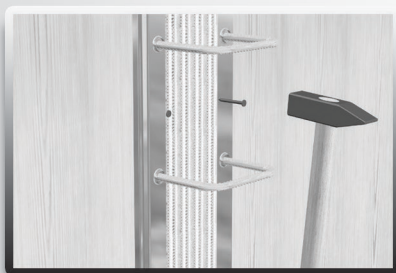
BWA connector should be nailed to the formwork through the perforation.
