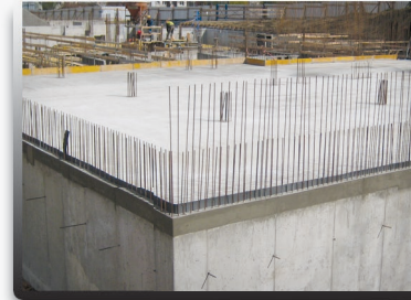
Fugenblech at contact area
